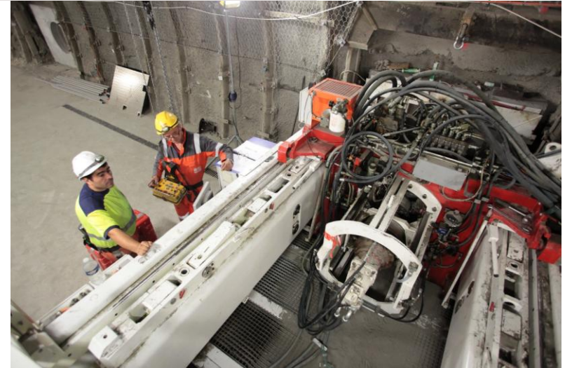
Boring of a HLW disposal cell (100 m) at the URL in July 2012 (Andra/CSM-Bessac)
